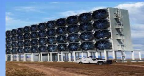
Direct Air Carbon Capture pulls ambient air through fans and into a process that separates then “captures” CO<sub>2</sub> which is then utilized or sequestered.
